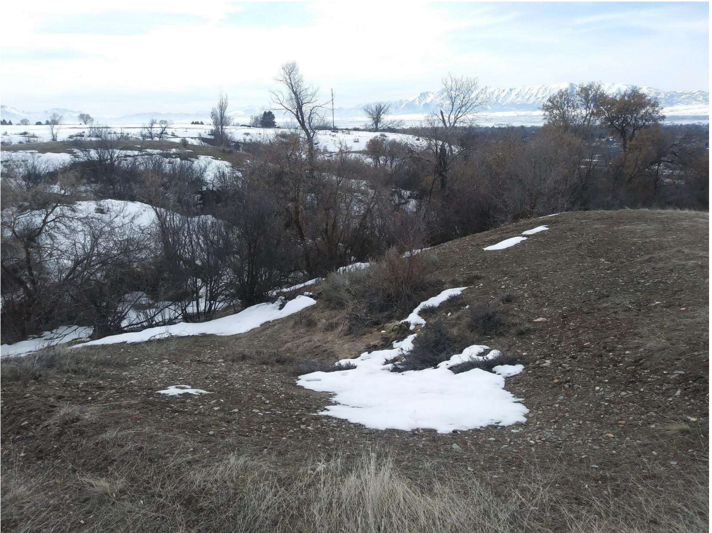
Photo 4 Ravines eroded into the slope on the northwest portion of the target property, looking southwest.
